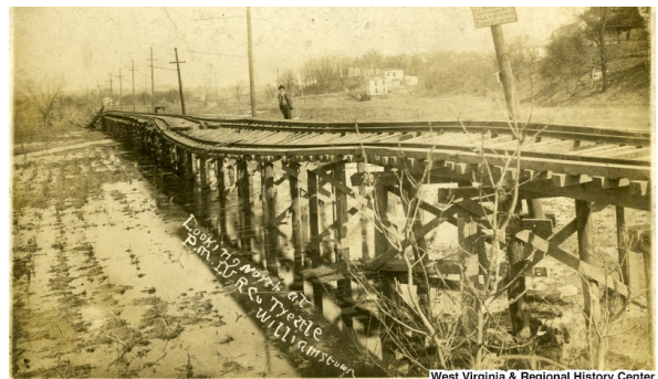
Looking north at Parkersburg Marietta Interurban Railroad Company Trestle, Williamstown, WV. View of a section of track, probably damaged by flood waters. 1913.
