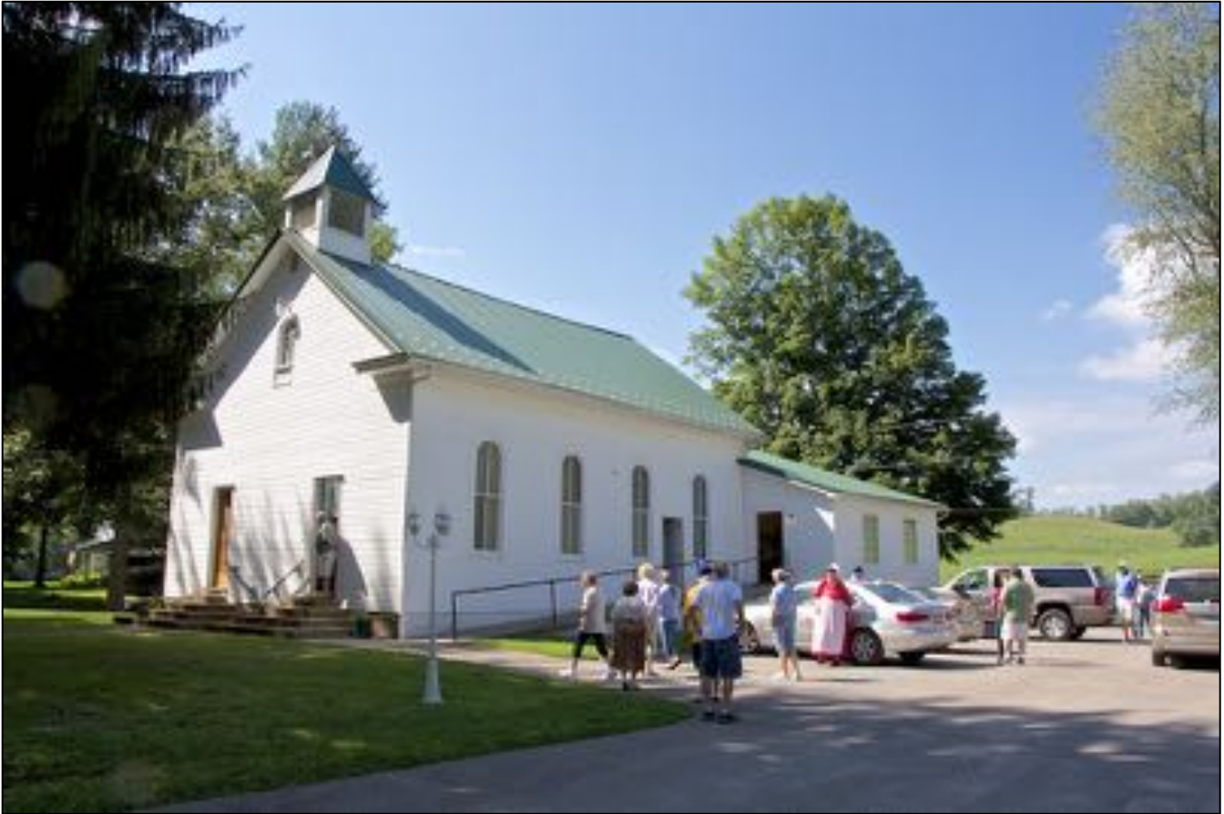
Bethany Baptist Church in Hall, WV. Erected in 1876.
