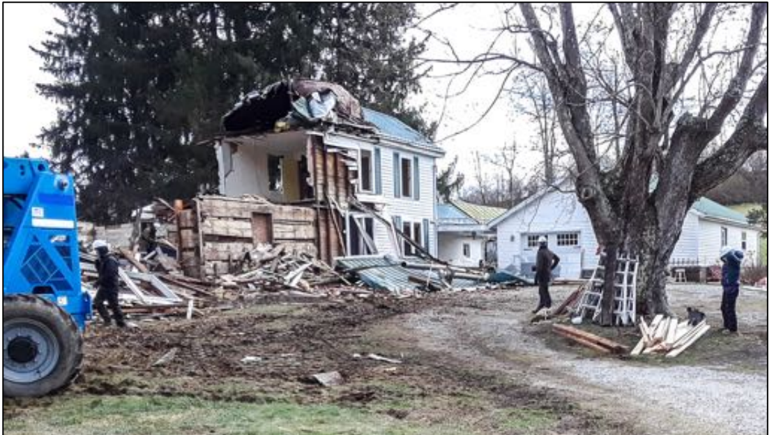
The Jacob Jay Jackson/Shaver House was demolished starting March 15, 2018. You can see a wall of the 27" poplar logs that Jacob Jay Jackson used in the original 1849 cabin.
