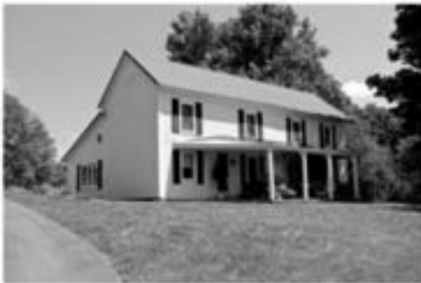
Doug and Ann Bush's home in sight of Henry Jackson Cemetery. One room contains Henry's cabin built in 1820.
